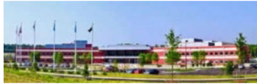
2010 Russell Knox Building completed with state of the art data center
